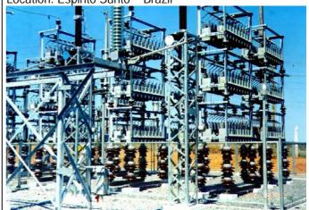
Description: One capacitor bank, 31.6MVAr - 132kV-60Hz, in star-connection with grounded neutral, including unbalance CT.
