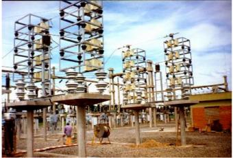
**Description:** One capacitor bank, 800kVAr - 55kV – 50Hz in bridge connection, with unbalance protection
